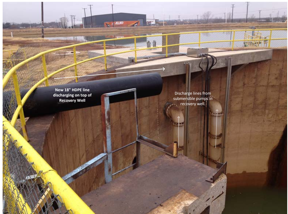
Photograph of new 18" HDPE line into the top of the recovery well.
