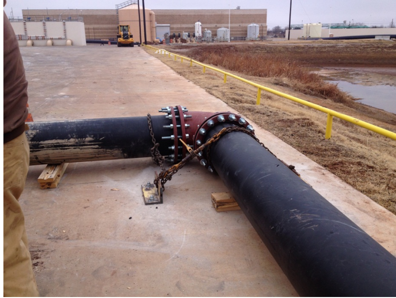
Photograph of new 18" HDPE line into the top of the recovery well.
