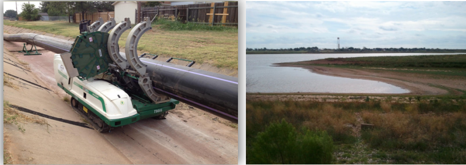
Figure 13-X: Left: Temporary DPR Pipeline Installation (Source: Nix, 2013) Right: Lake Arrowhead Levels in 2013 (Source: Nix, 2013)
