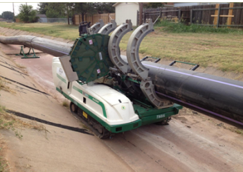
Figure A.6-2 Temporary DPR Pipeline Installation (Photo credit: XX )
